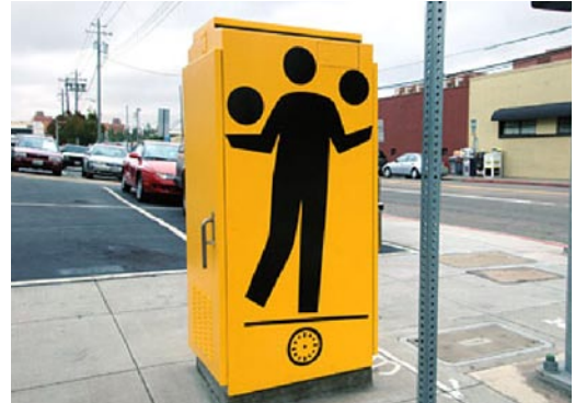
Utility box designed by Seyed and students
